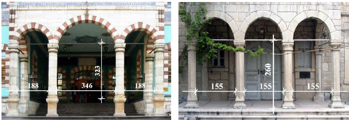
Figure 5. (Left) Kütahya government palace, entrance columns; (Right) Kalecik government palace, entrance columns (Source: Ö. Aydın archive).
