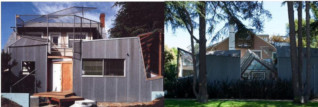
Figure 5. Gehry House, Frank Gehry, Californiya, 1978 (URL-7).
