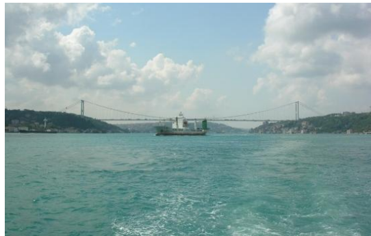
Figure-13. The Bosphorus Bridge.
