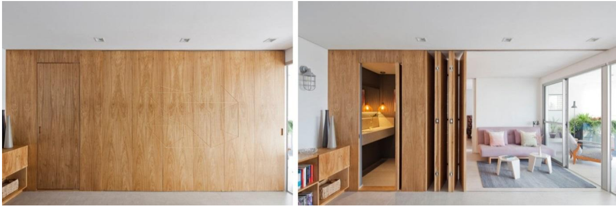
Figure.5. Example of a Full Divider Opened by Folding
